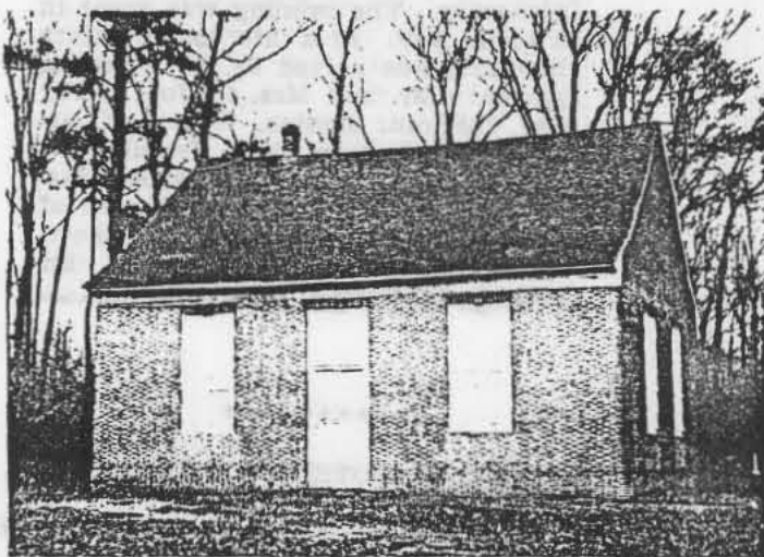
St. Martin's Church ... restoration plans aided by $40,000 grant.
